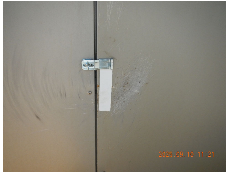
4. Repaired meter shed door handle.
