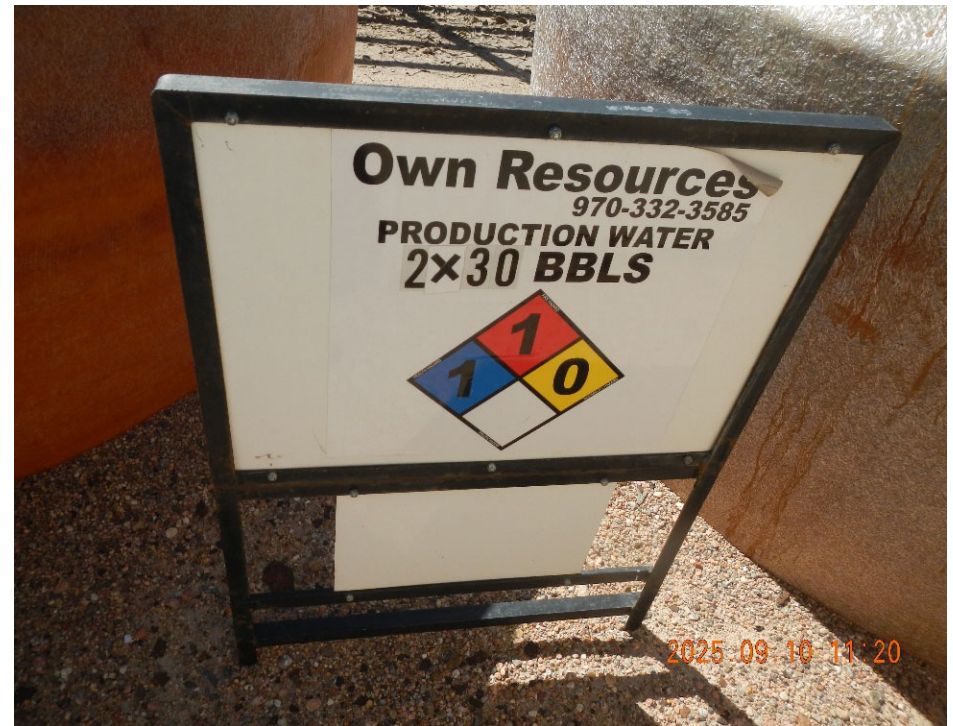
2. New Content/Quantity/Hazard sign at produced water tanks.
