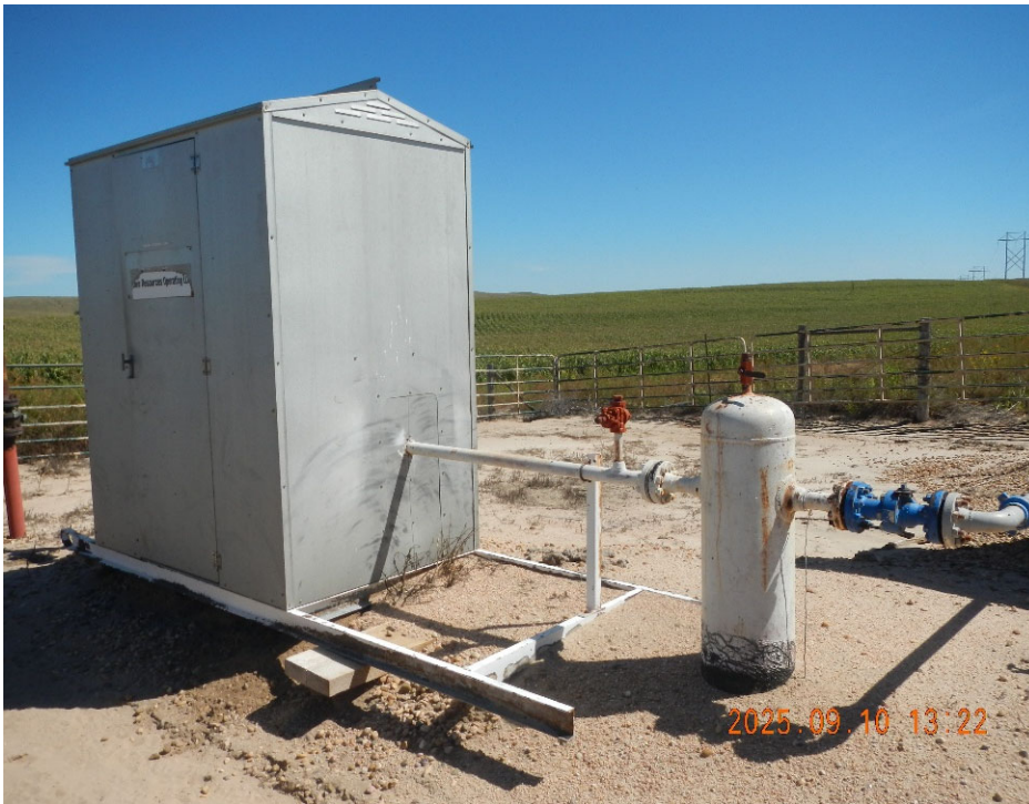
5. View of abandoned flowline equipment.
