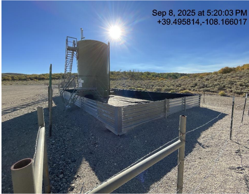
Photo # 7124 Tank battery lacks required signage
