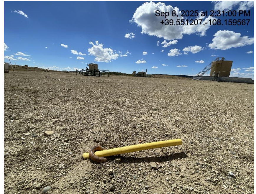
Photo # 6808 Same improperly marked deadman
