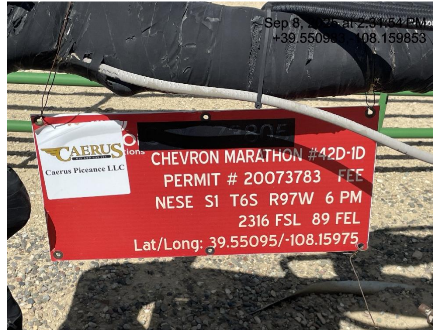
Photo # 6806 Wellhead sign has previous operators name
