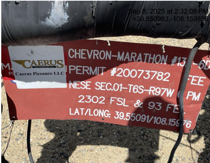
Photo # 6805 Wellhead sign has previous operators name
