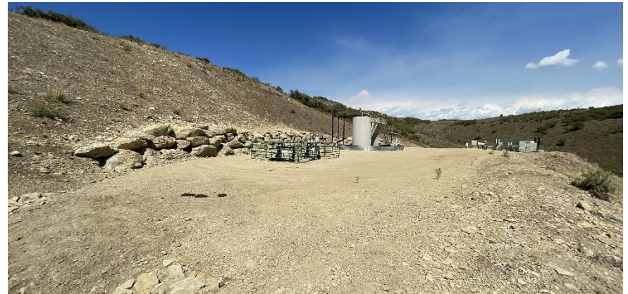
South East corner of location.
