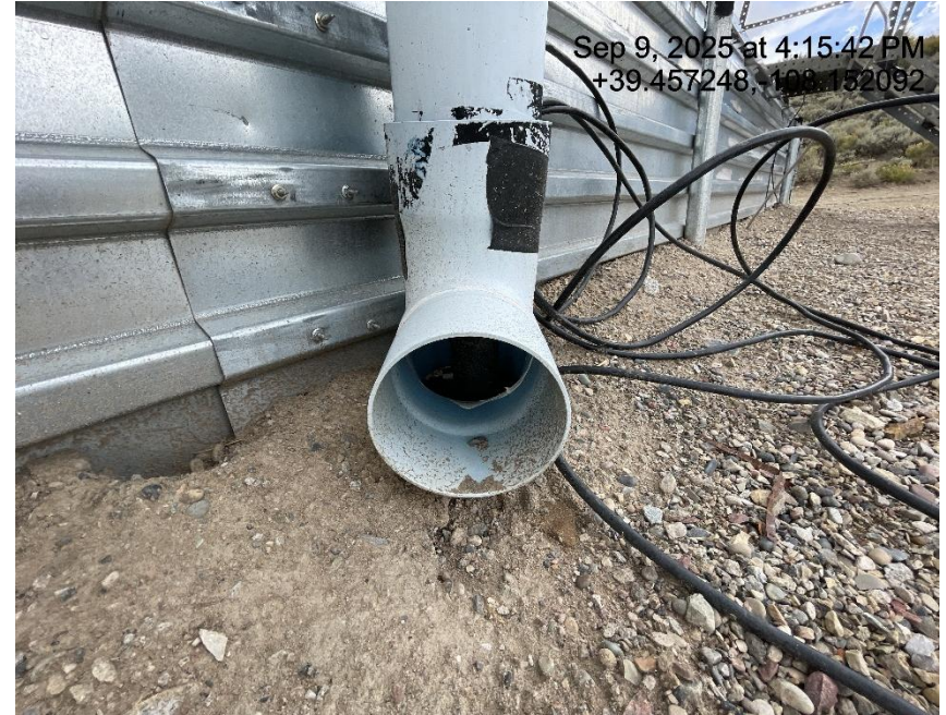
Photo # 7780 Flowline heating insulation open ended /wildlife hazard/available for entry by wildlife
