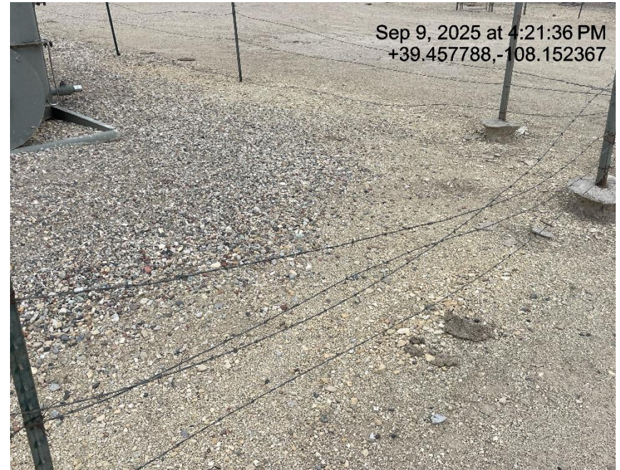
Photo # 7782 Barbed wire fence around separators needs maintenance/wildlife hazard
