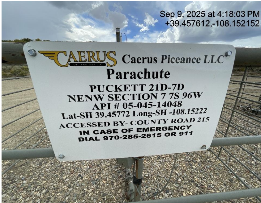
Photo # 7789 Wellhead sign has previous operators name
