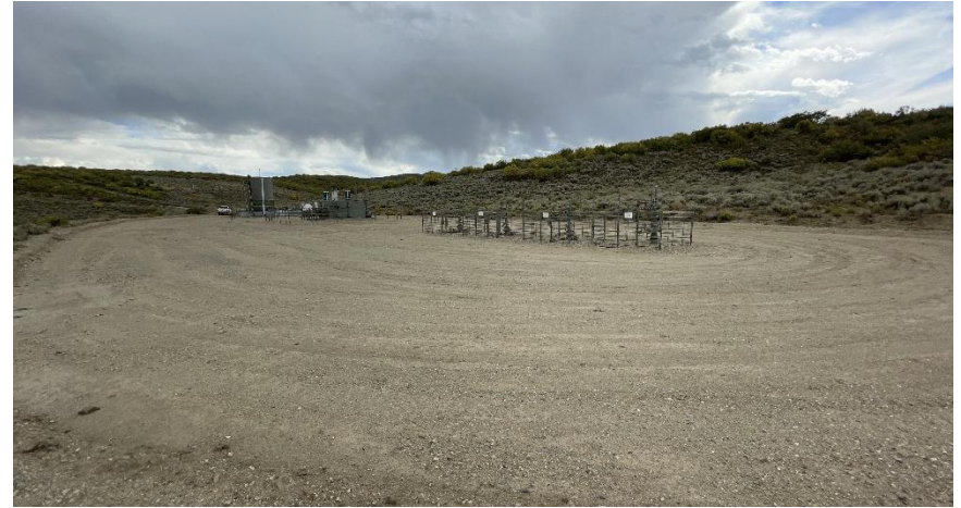
North East corner of location.
