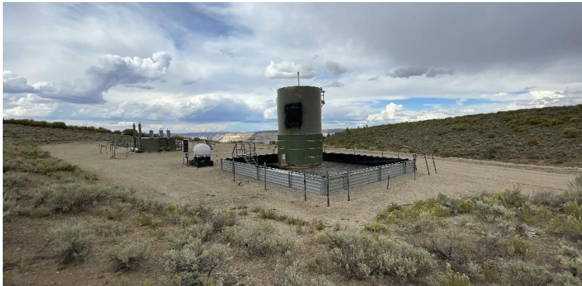
South West corner of location.
