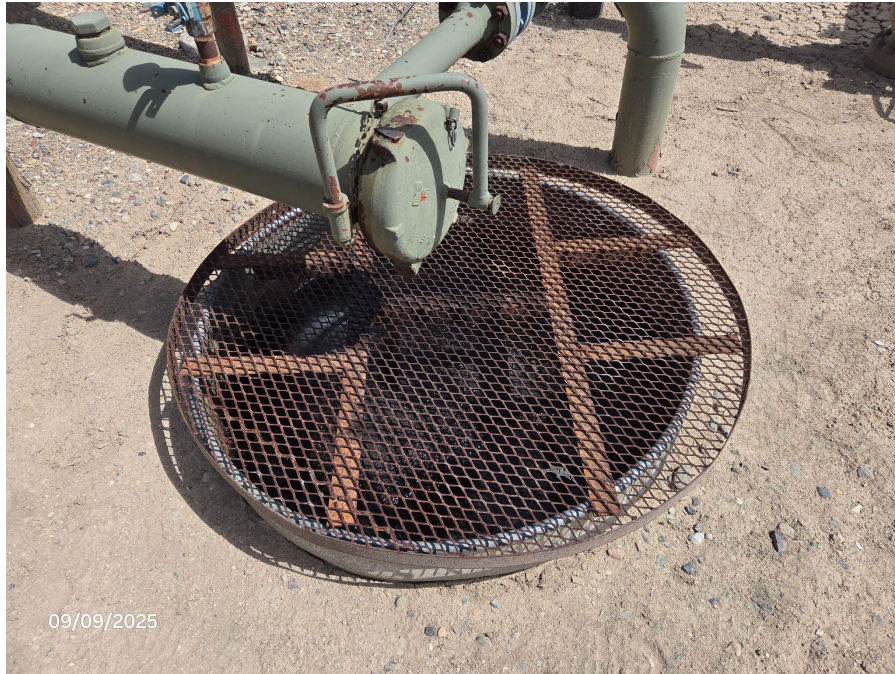
Photo 5: Photo taken from pipe equipment on the northeast end of the Location. Photo shows spill within containment.
