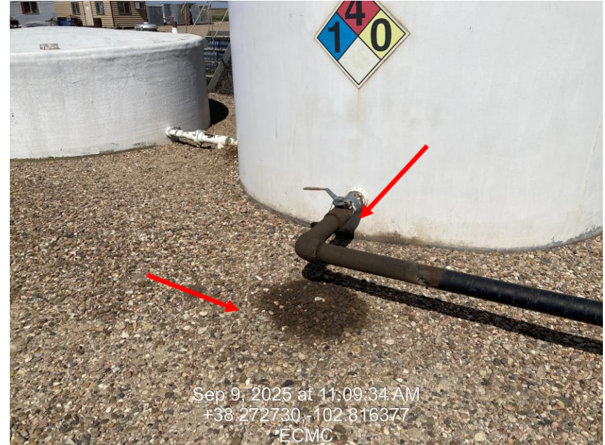
Photo 6 – Leak on 90* elbow, impacted soils
