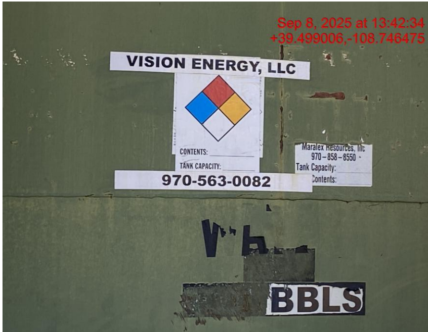
Labels Missing Required Information – Photo #00629
