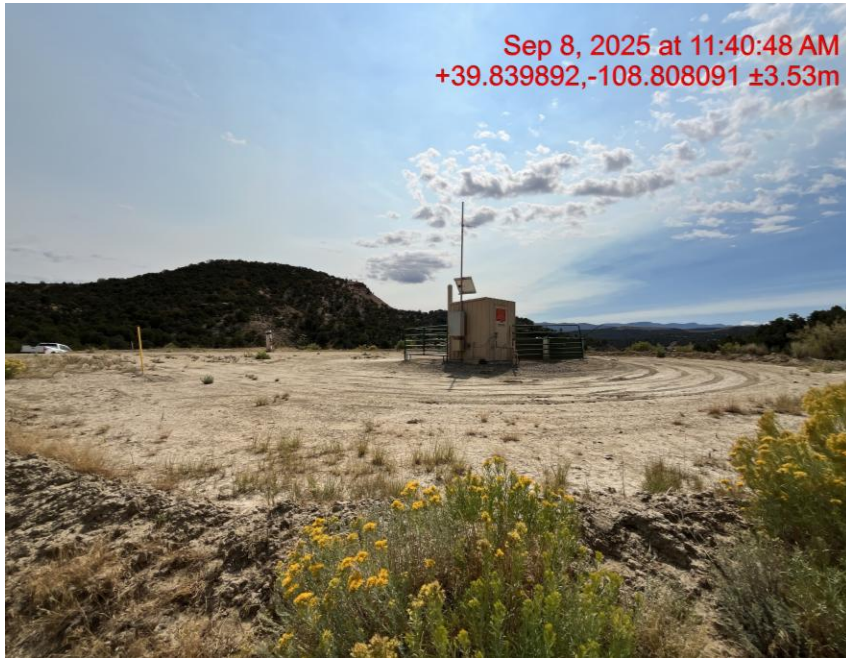
Photo # 3015 NW corner of location
