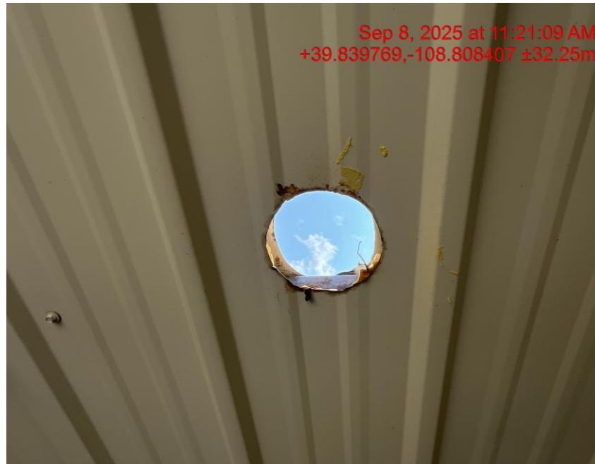
Photo # 2993 Hole in meter house open to wildlife/available for entry by wildlife
