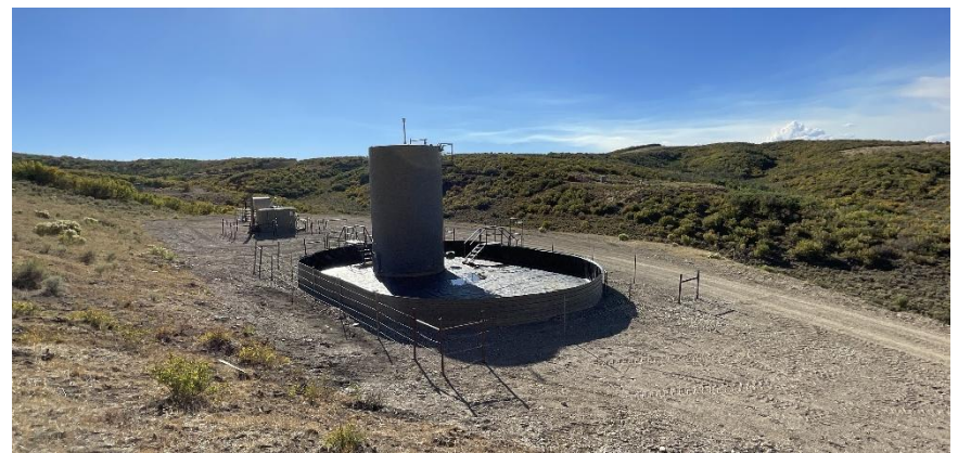
South East corner of location.
