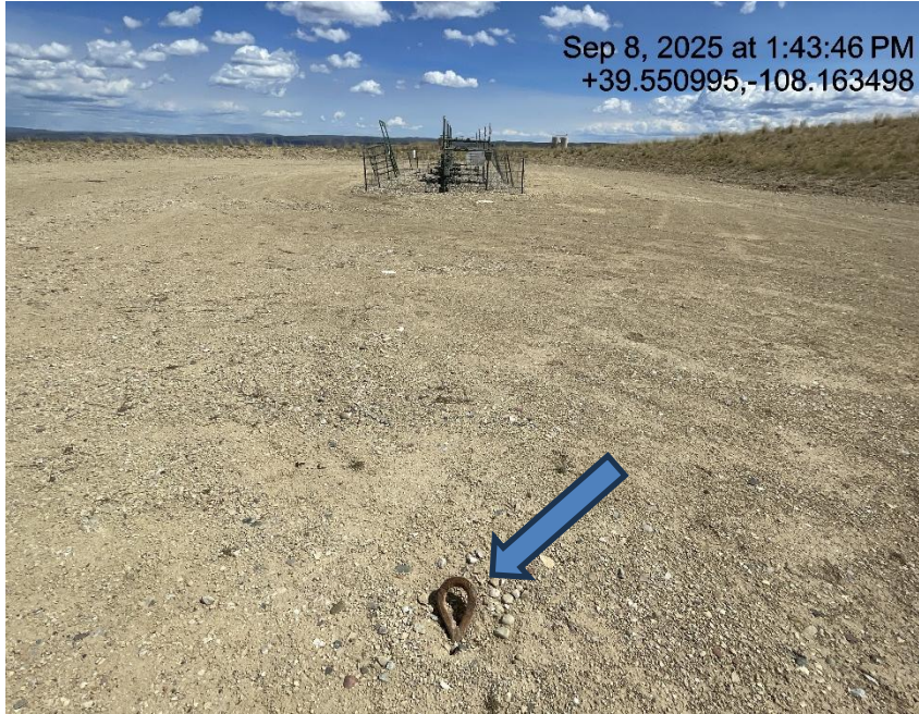
Photo # 6642 Unmarked deadman
