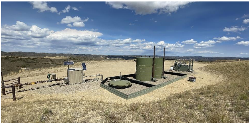
South West corner of location.
