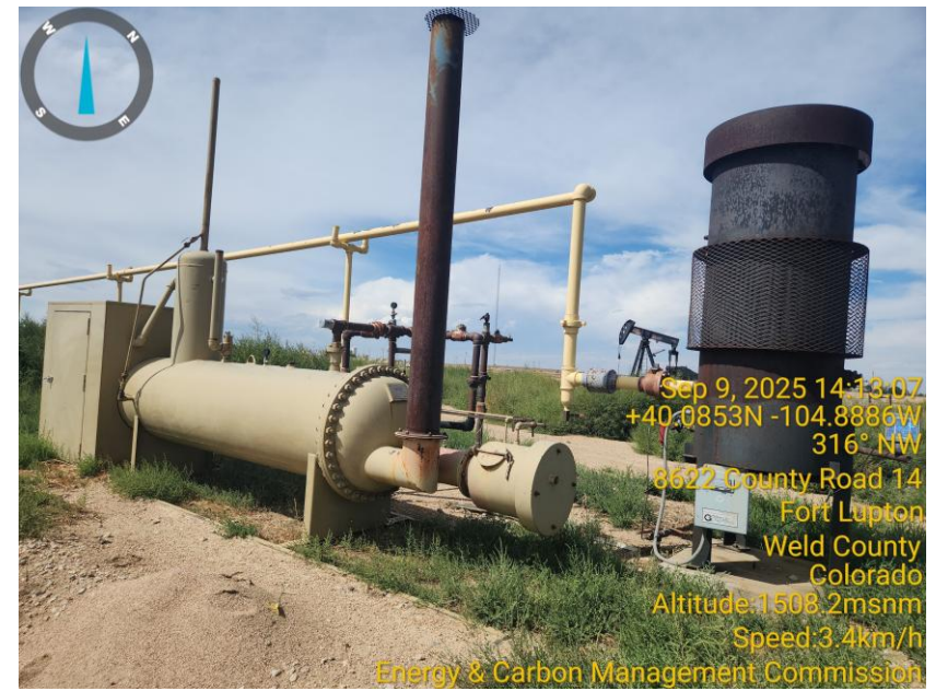
Photo 2 ECD, Horizontal Heated Separator.
