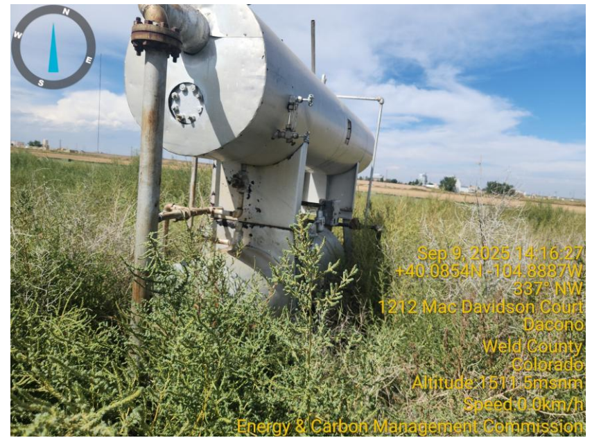
Photo 12 Horizontal separator is overrun with vegetation.
