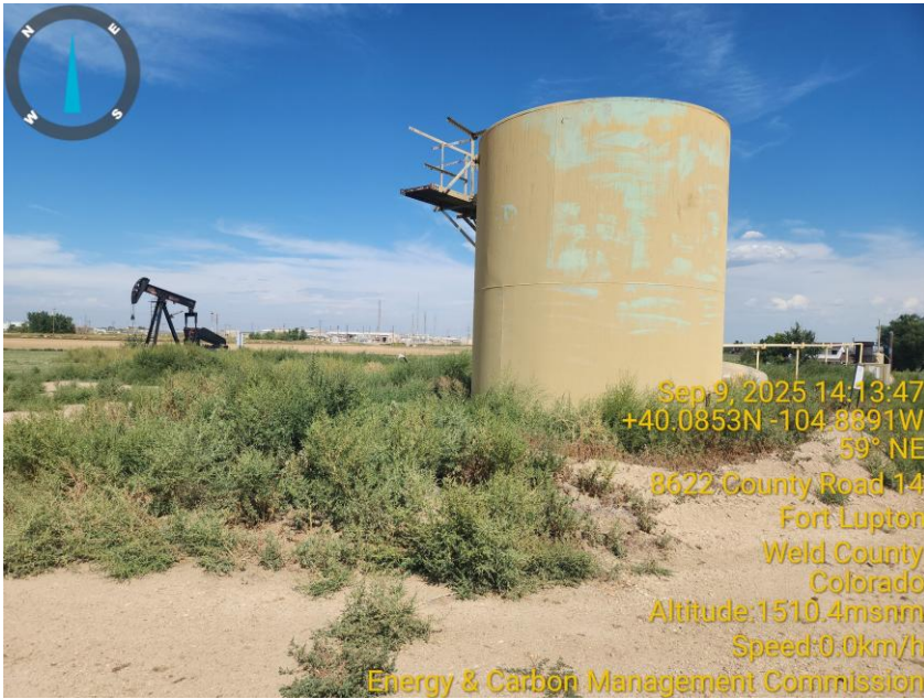
Photo 5 Tank Battery is overrun with vegetation .
