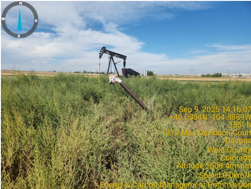
Photo 11 Unmarked flow line is overrun with vegetation.
