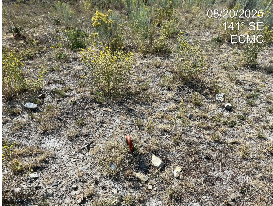
Photo 5. Photo taken of one of the four remaining guy line anchors still left on Location.
