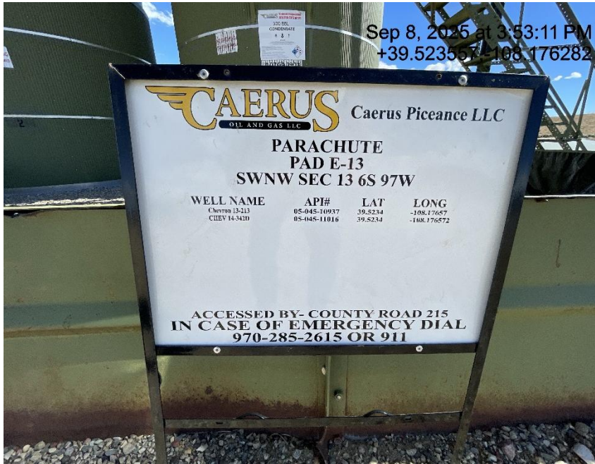
Photo # 6893 Battery sign has previous operators name
