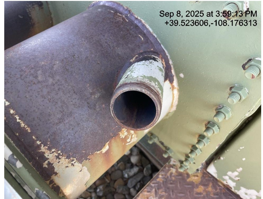
Photo # 6890 Open ended pipe on fire tube/wildlife hazard
