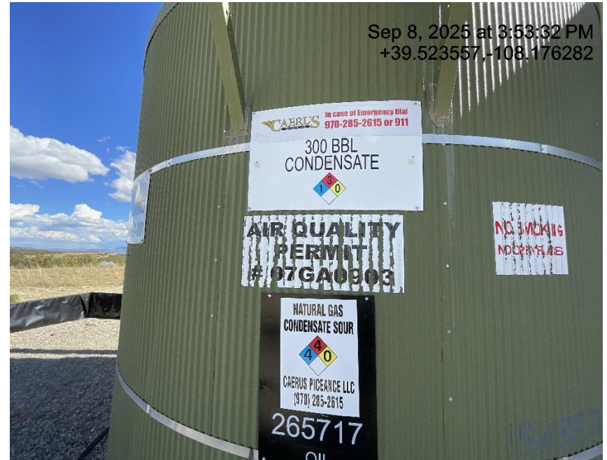
Photo # 6896 Tank labels have previous operators name
