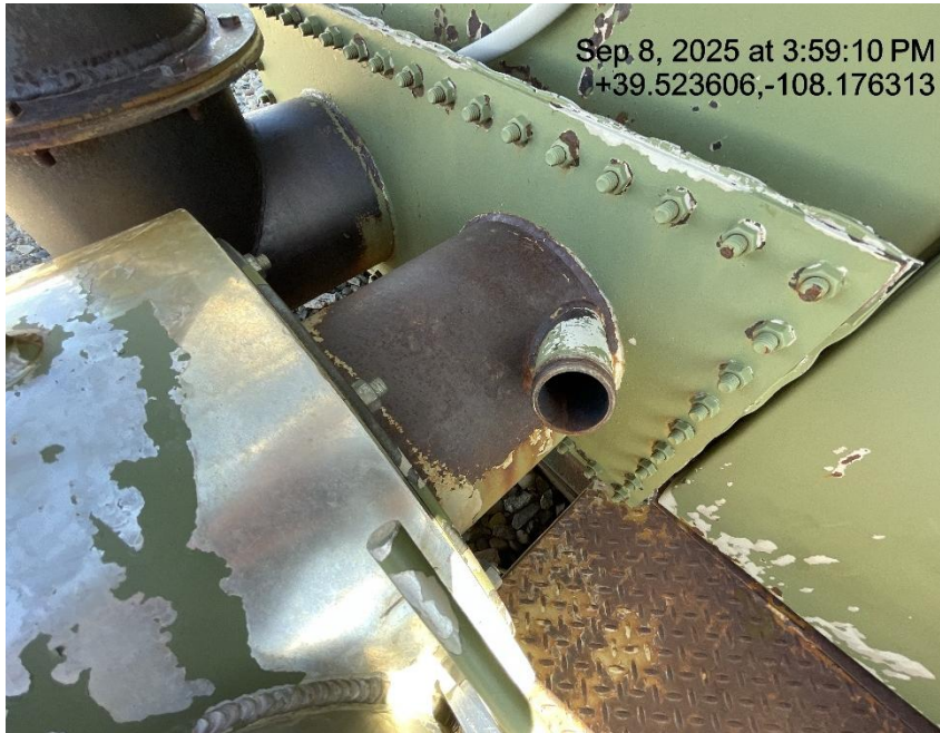
Photo # 6889 Open ended pipe on fire tube/wildlife hazard
