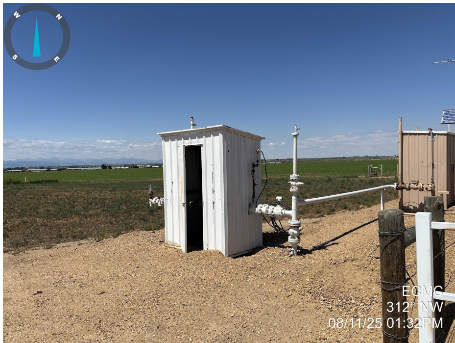
Photo 7. Photo taken of the eastern portion of the tank battery location, facing northwest. Photo illustrates that midstream equipment remains on the location.
