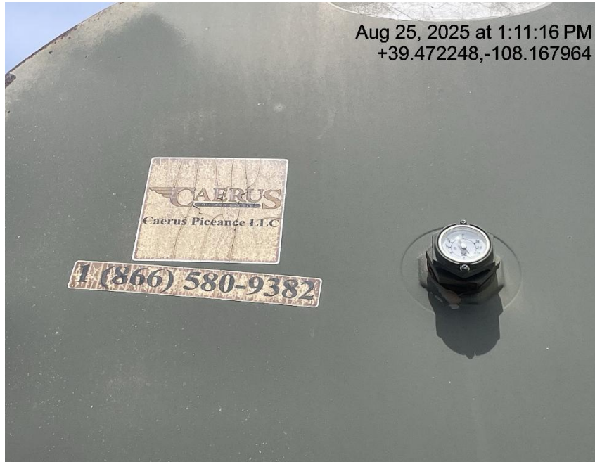
Photo # 3870 Tank label has previous operators name
