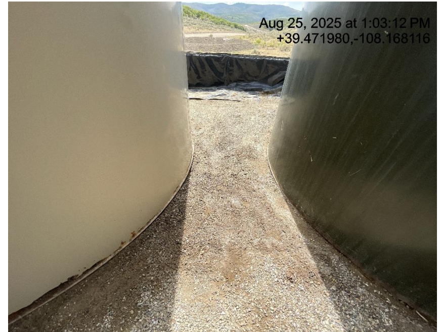
Photo # 3875 Staining in secondary containment
