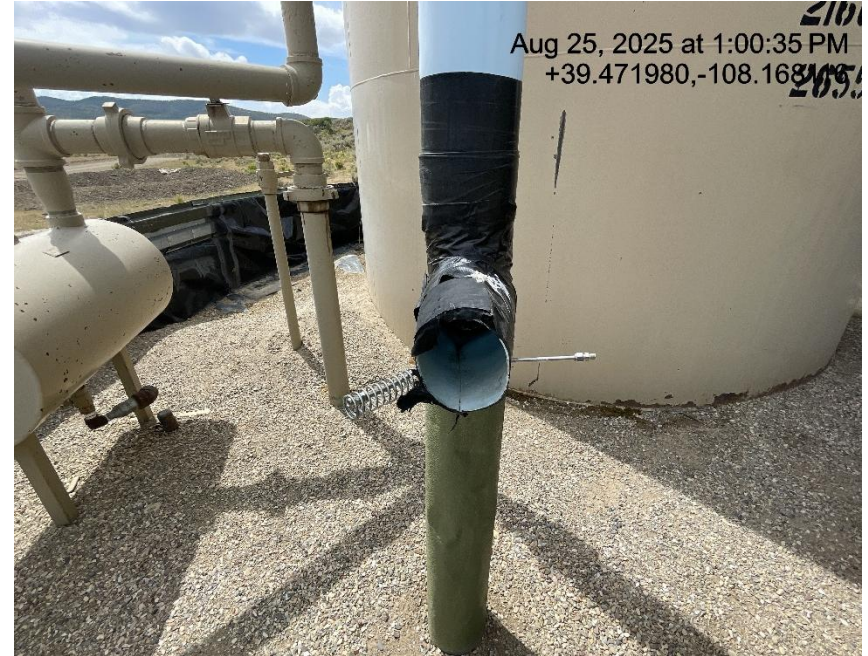
Photo # 3861 Flowline heating insulation open ended /wildlife hazard/available for entry by wildlife
