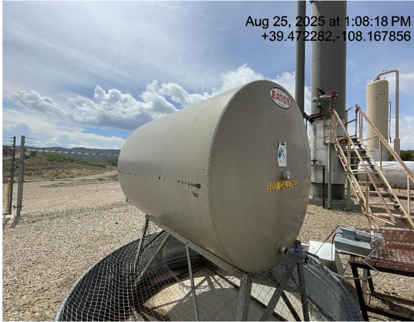
Photo # 3854 Chemical tank lacks required labeling
