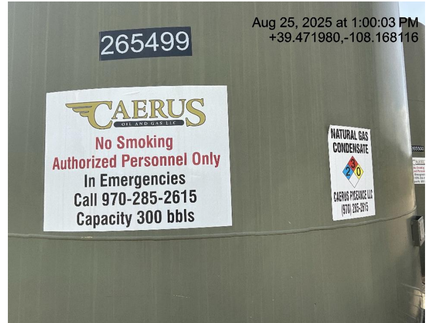
Photo # 3871 Tank label has previous operators name
