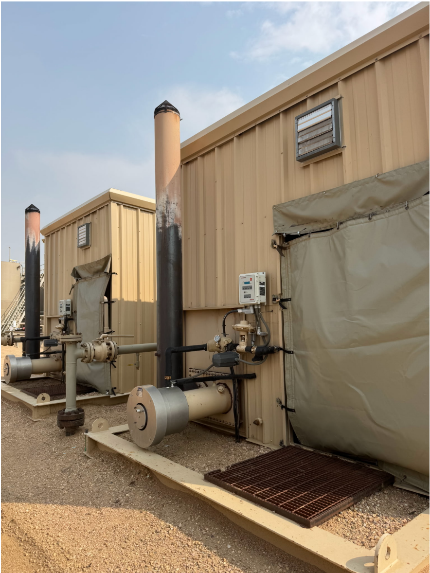
Wildlife screen installed.
