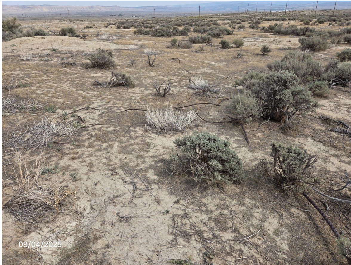
Photo 2: Cable/debris remaining on the Location.
