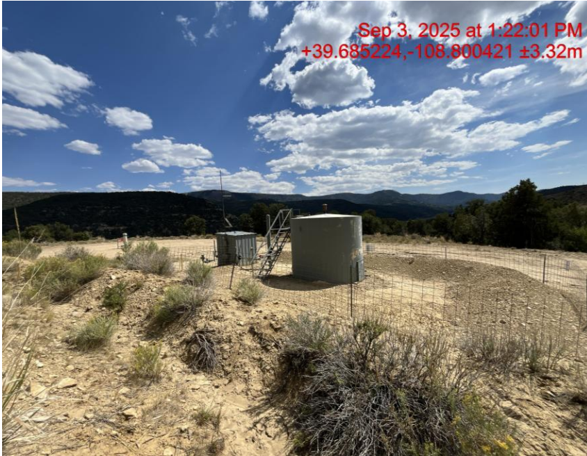
Photo # 2869 NW corner of location
