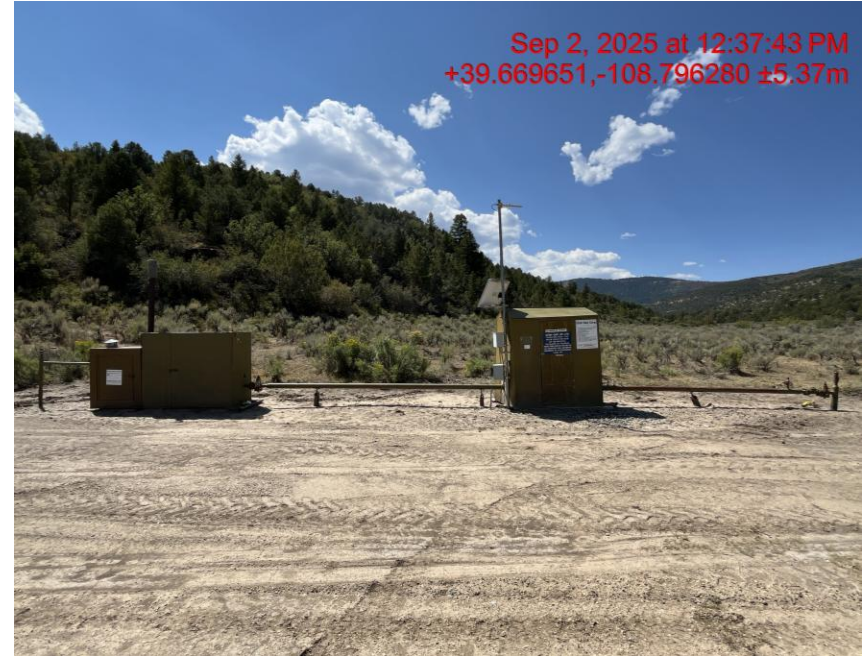
Photo # 2819 Location – Tank battery has been removed
