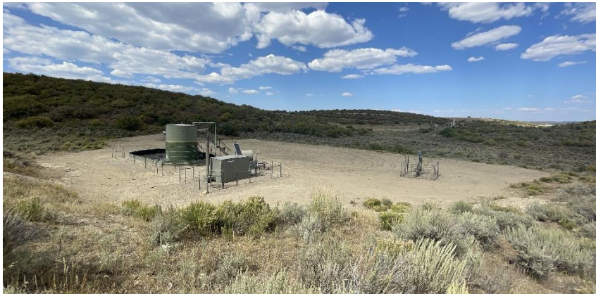
South West corner of location.
