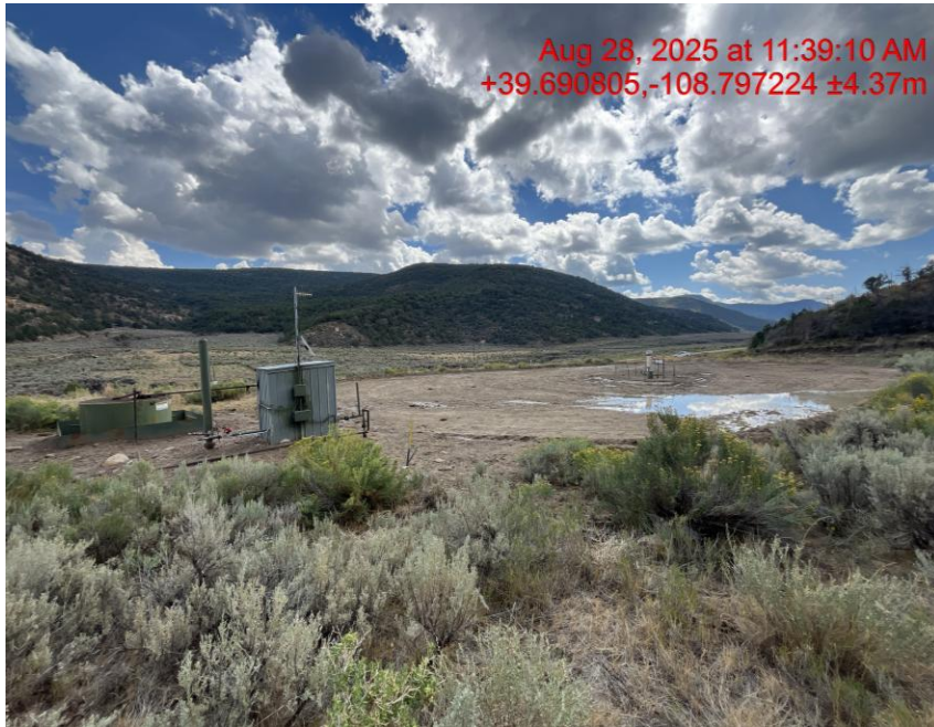
Photo # 2748 NW corner of location
