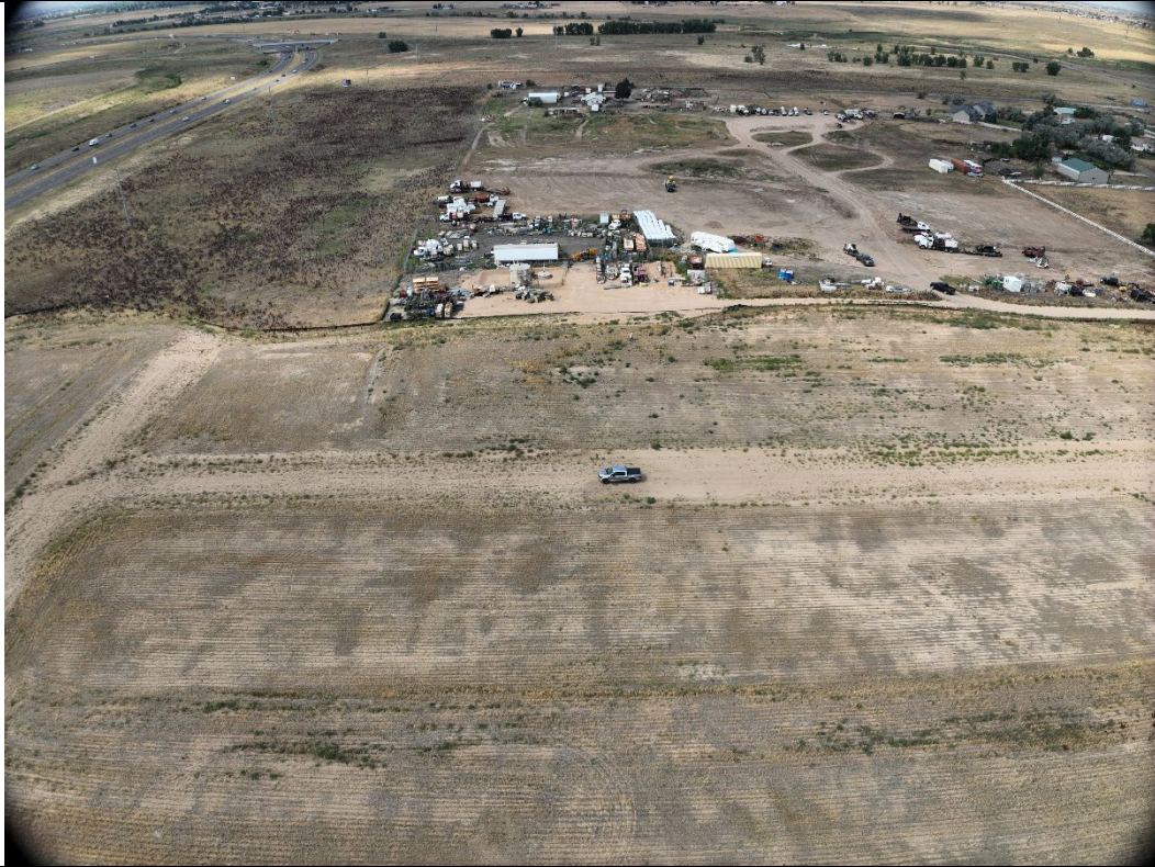
In View – Tank Battery (Loc ID 452734 ), Access Road, Flowline
