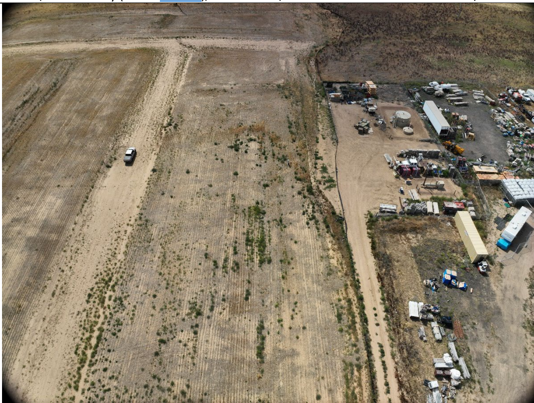
In View – Well, Tank Battery (Loc ID 452734 ), Access Road, Flowline WEST – 39.892573 / -104.758298
