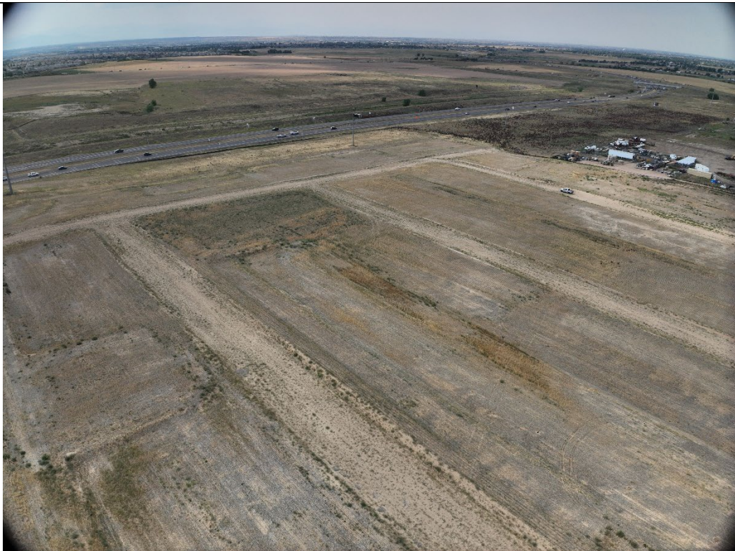
In View – Well, Tank Battery (Loc ID 452734 ), Access Road, Flowline
