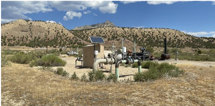
South West corner of location.
