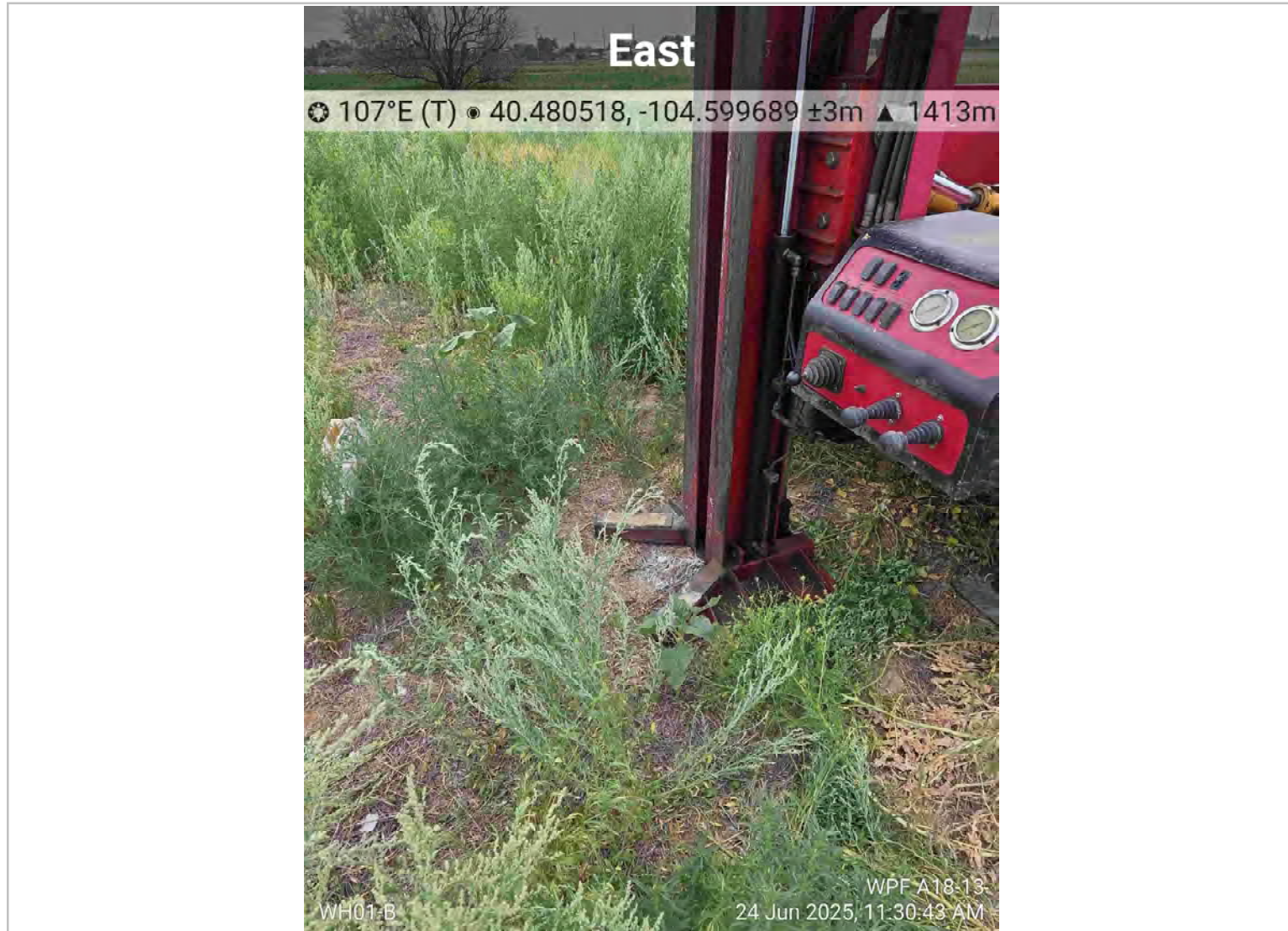
Soil Boring WH01-B: View East
