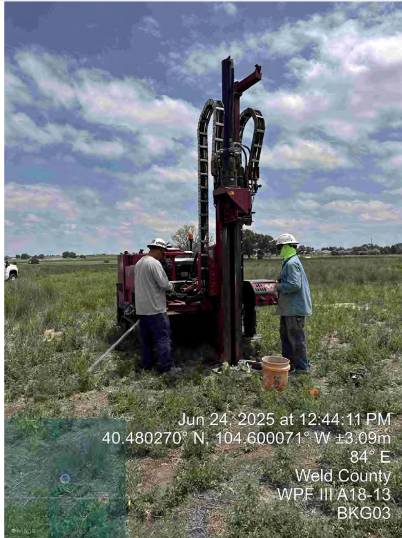
Soil Boring BKG03: View East
