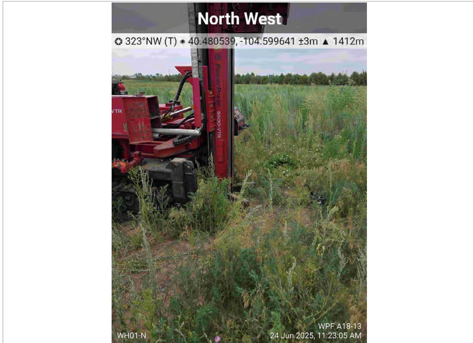
Soil Boring WH01-N: View Northwest
