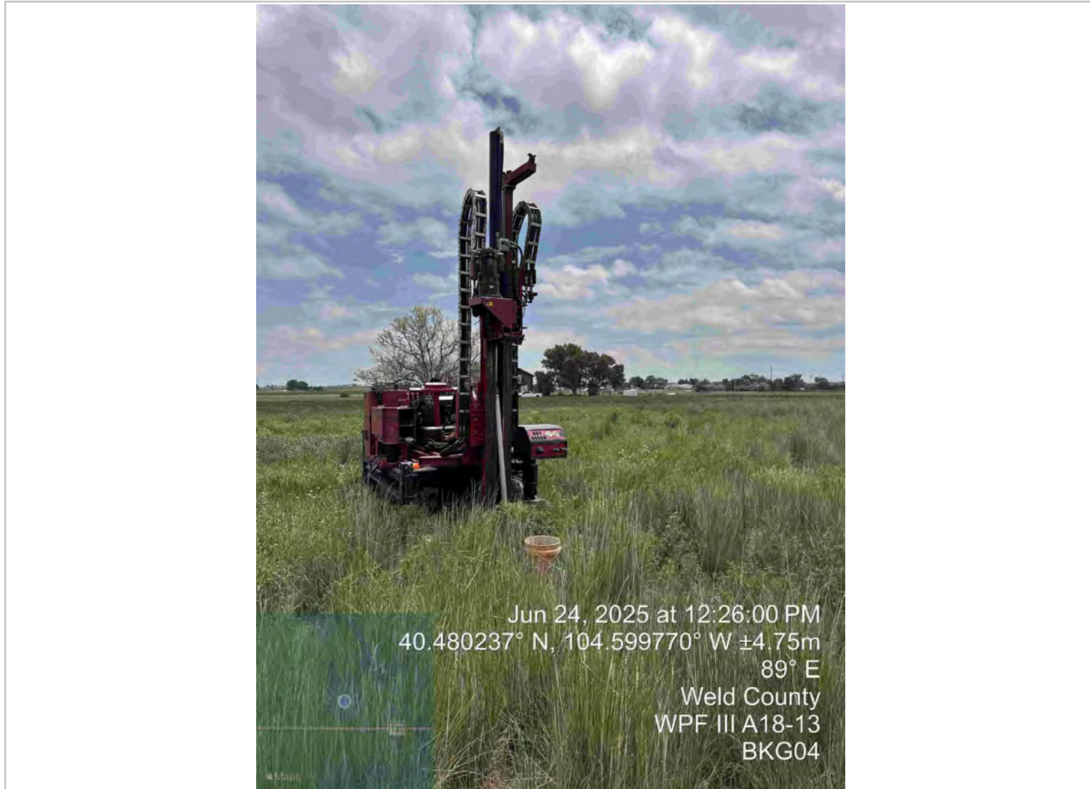
Soil Boring BKG04: View East
