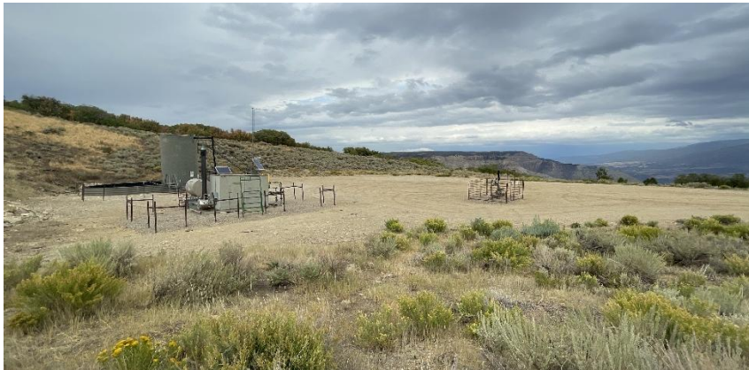
South West corner of location.
