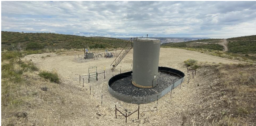
South West corner of location.
