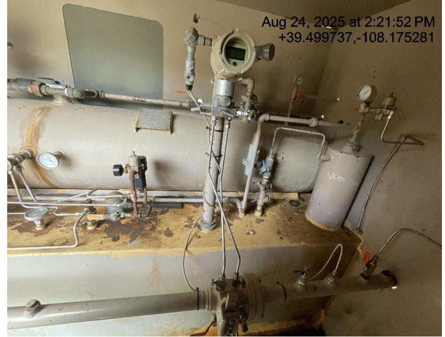
Photo # 3184 Meter calibration info not conspicuously posted
