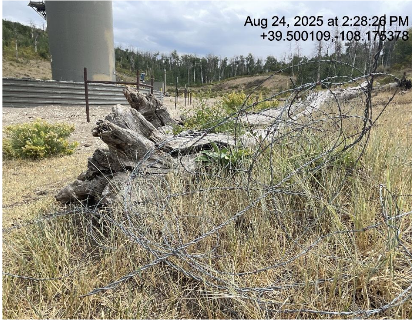
Photo # 3195 Loose barbed wire/wildlife hazard
