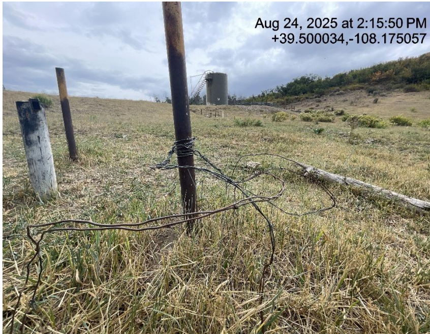
Photo # 3187 Loose barbed wire/wildlife & personnel hazard
