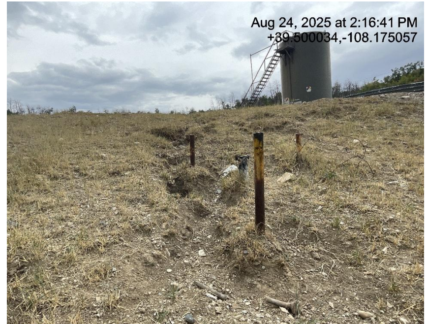
Photo # 3197 Erosion & transport of sediment off location /insufficient BMP's
