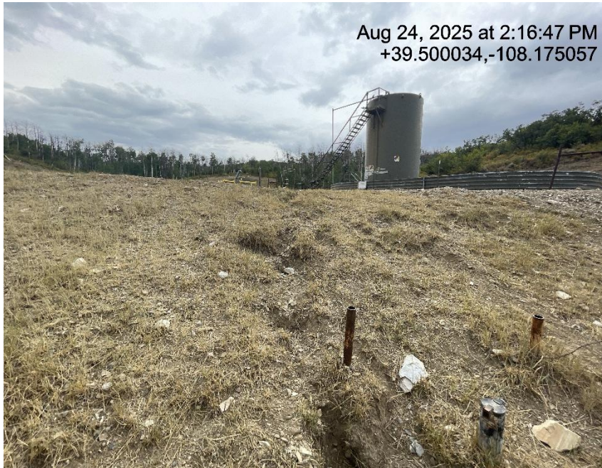
Photo # 3196 Erosion & transport of sediment off location /insufficient BMP's
