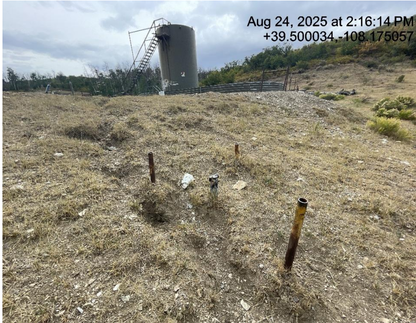
Photo # 3198 Erosion & transport of sediment off location /insufficient BMP's
