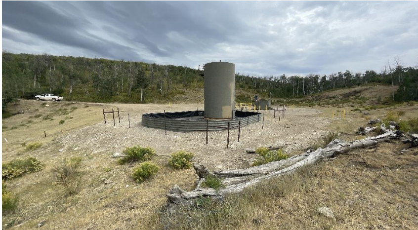
North West corner of location.
