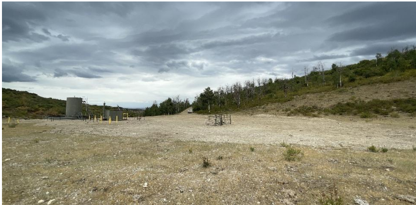
South West corner of location.
