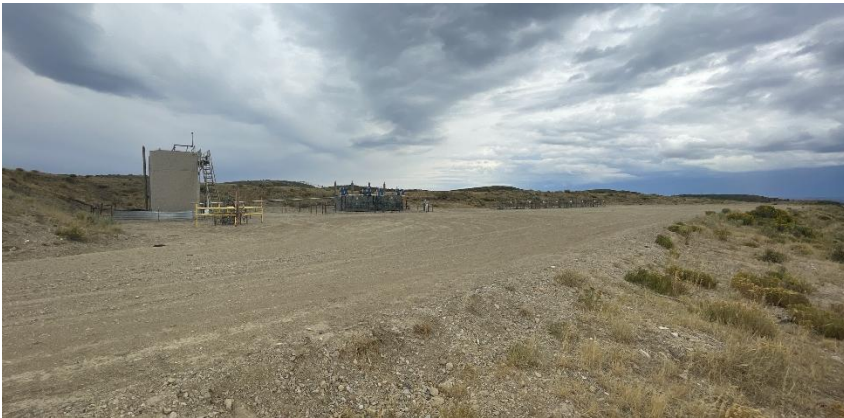
South West corner of location.
