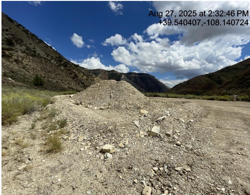
Photo # 4631 Soil stockpile with dirt berm BMP
