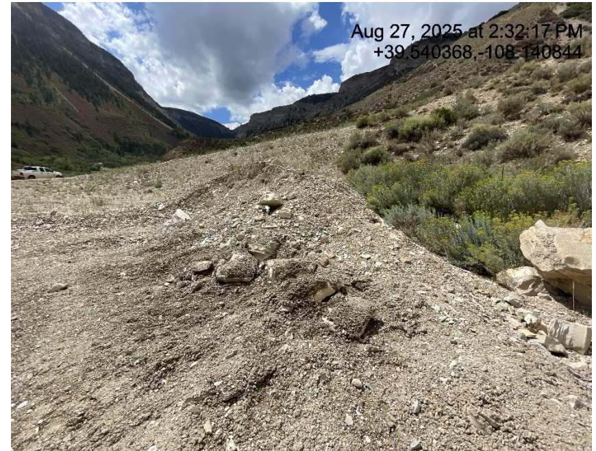
Photo # 4630 Stockpiled soils lack BMP's
