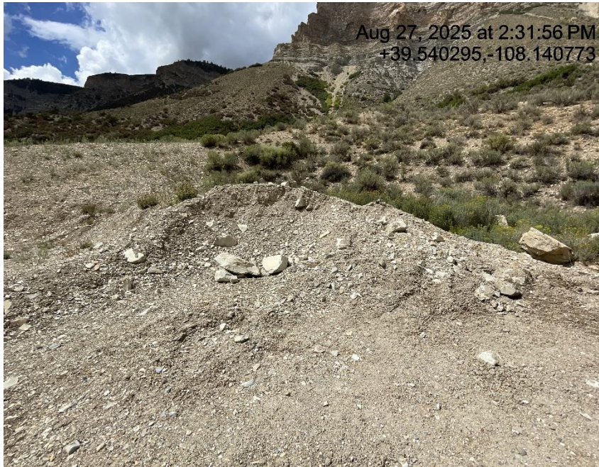
Photo # 4629 Stockpiled soils lack BMP's
