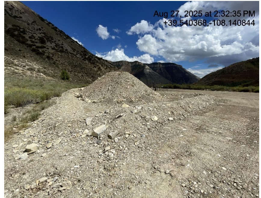
Photo # 4632 Soil stockpile with dirt berm BMP
