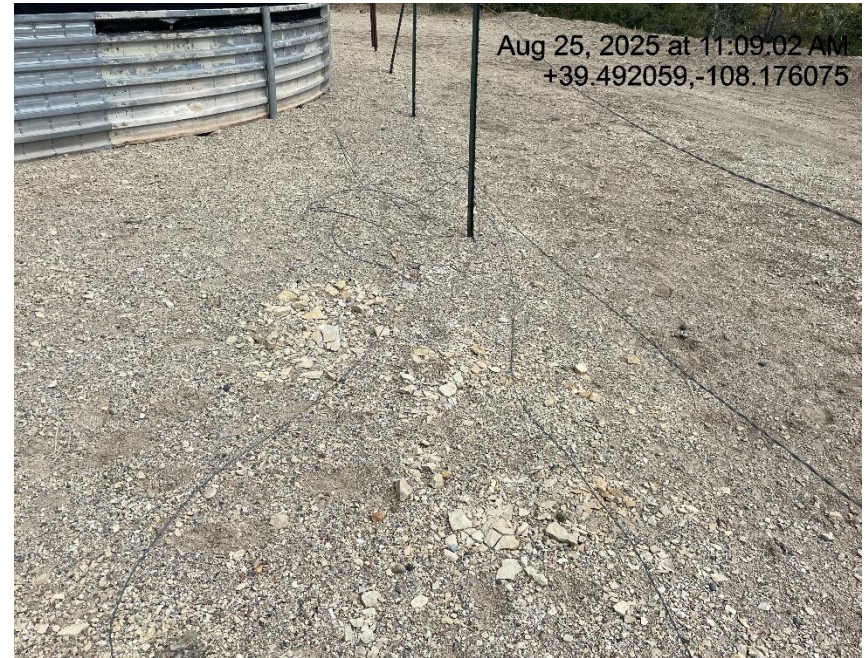
Photo # 3459 Fencing needs maintenance/wildlife hazard
