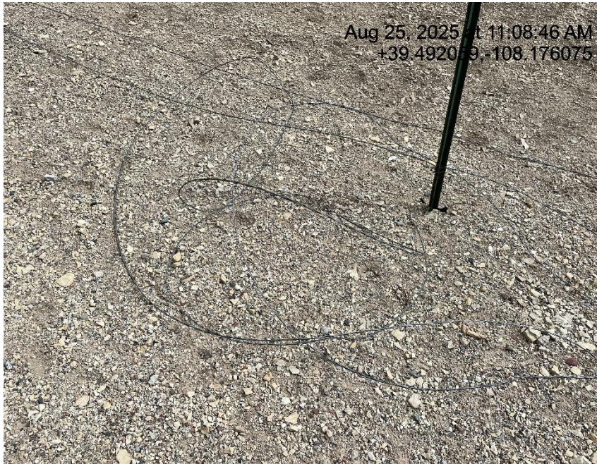
Photo # 3458 Fencing needs maintenance/wildlife hazard
