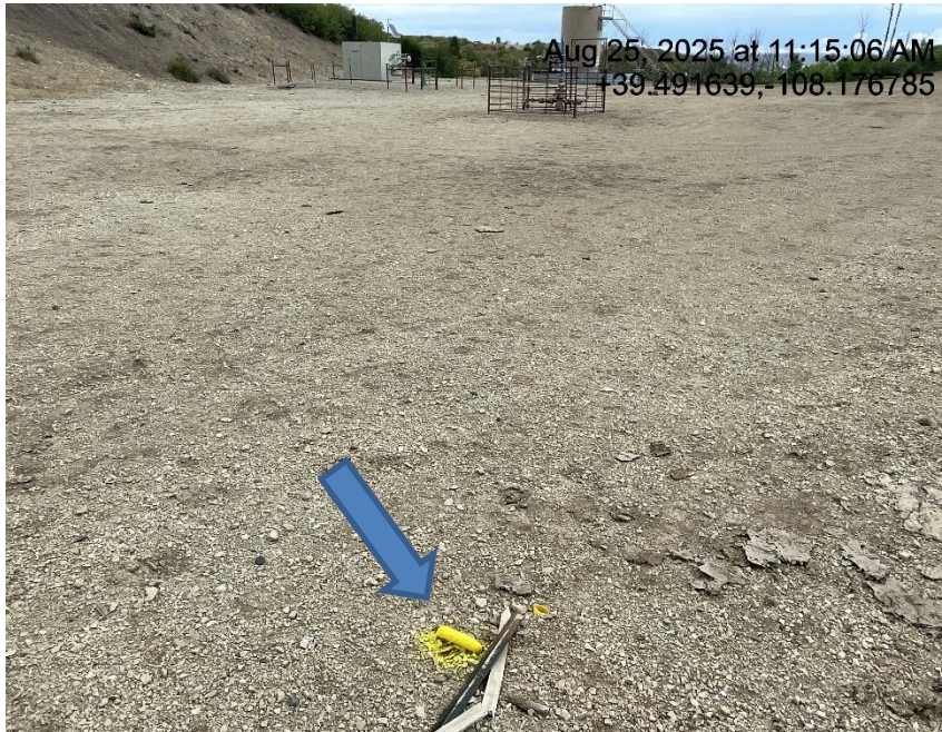
Photo # 3462 Unmarked deadman
