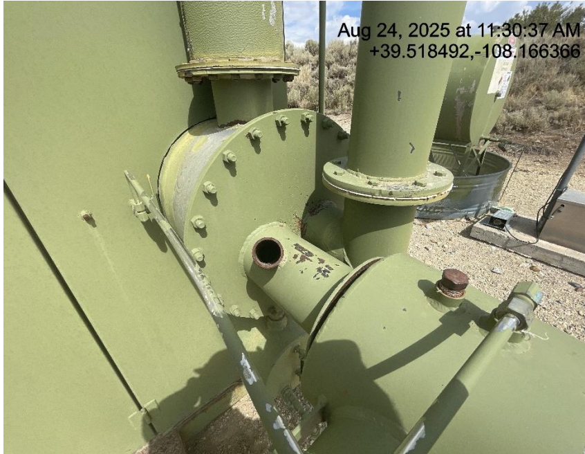
Photo # 2786 Open ended piping on fire tube/wildlife hazard
