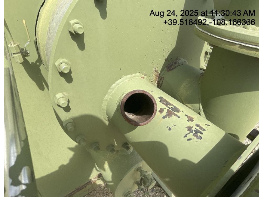
Photo # 2787 Open ended piping on fire tube/wildlife hazard
