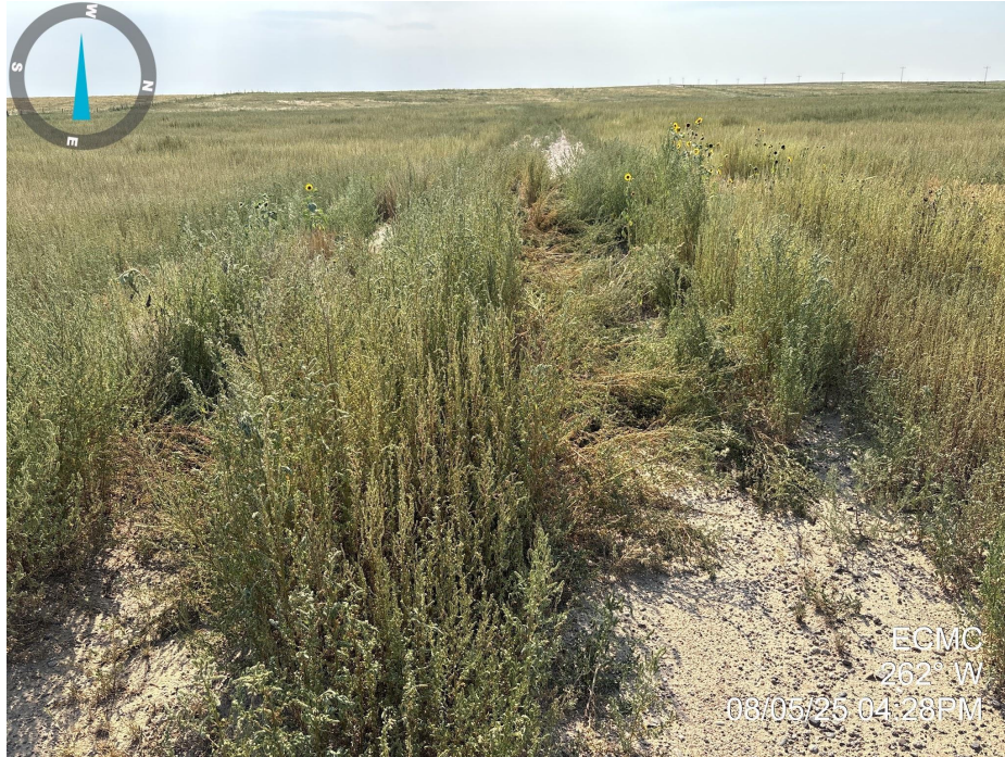
Photo 5. Photo taken of the access road to the well location, facing west, towards the location. Photo illustrates that the access road does not meet Rule 1004 standards as bare ground, gravel, and weedy annual vegetation were observed across the road.
