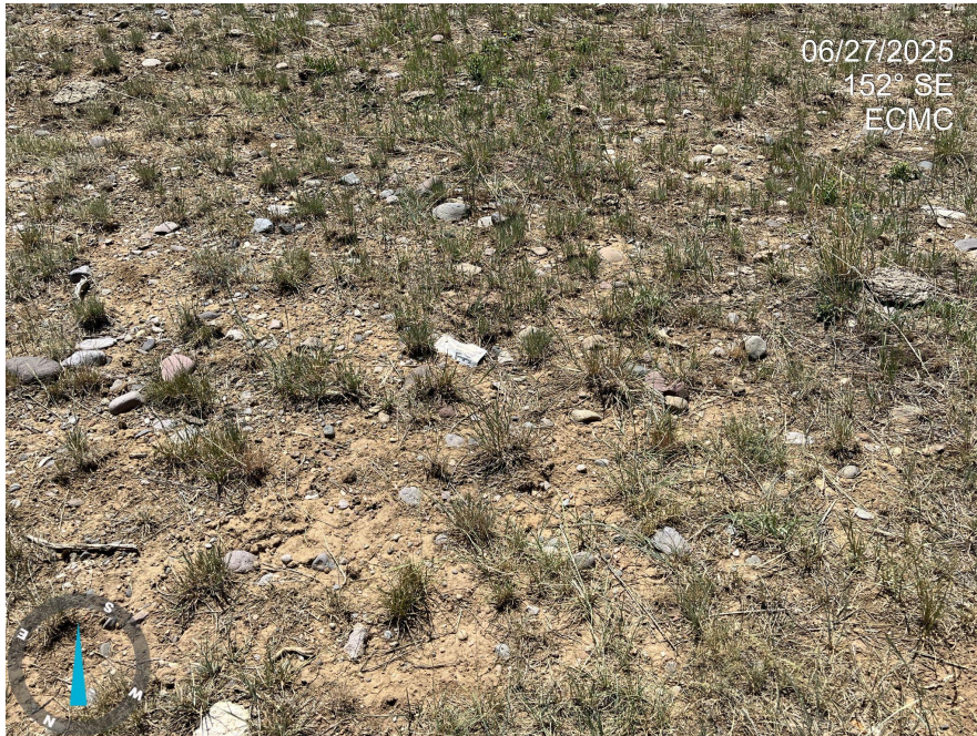
Photo 5. Photo taken illustrating that gravel has not been removed, and compaction alleviation has not occurred.
