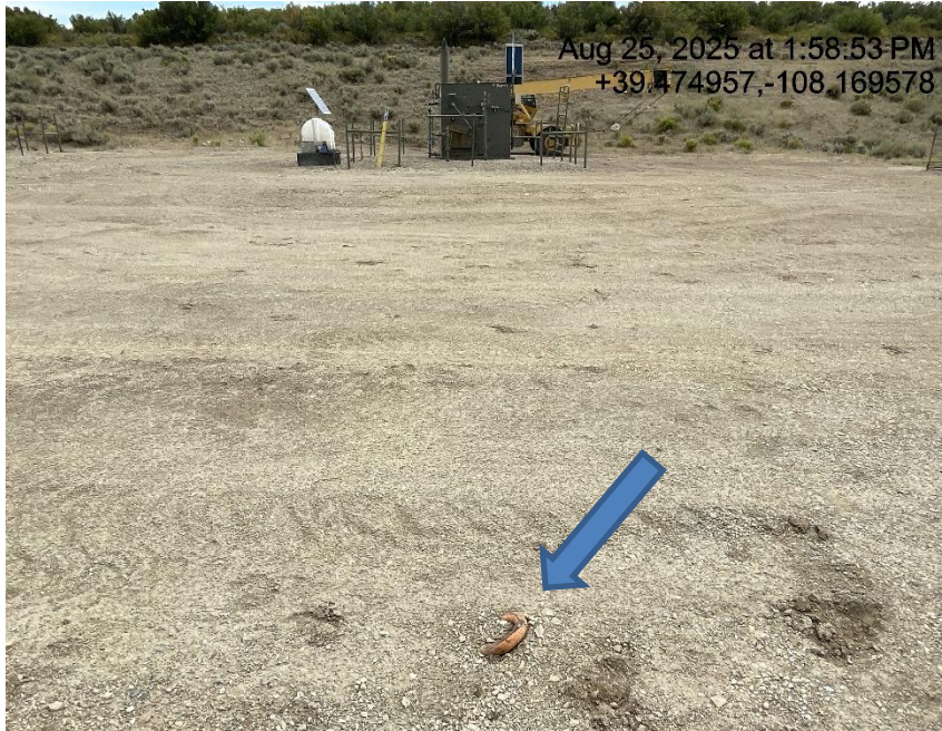
Photo # 4026 Same unmarked deadman
