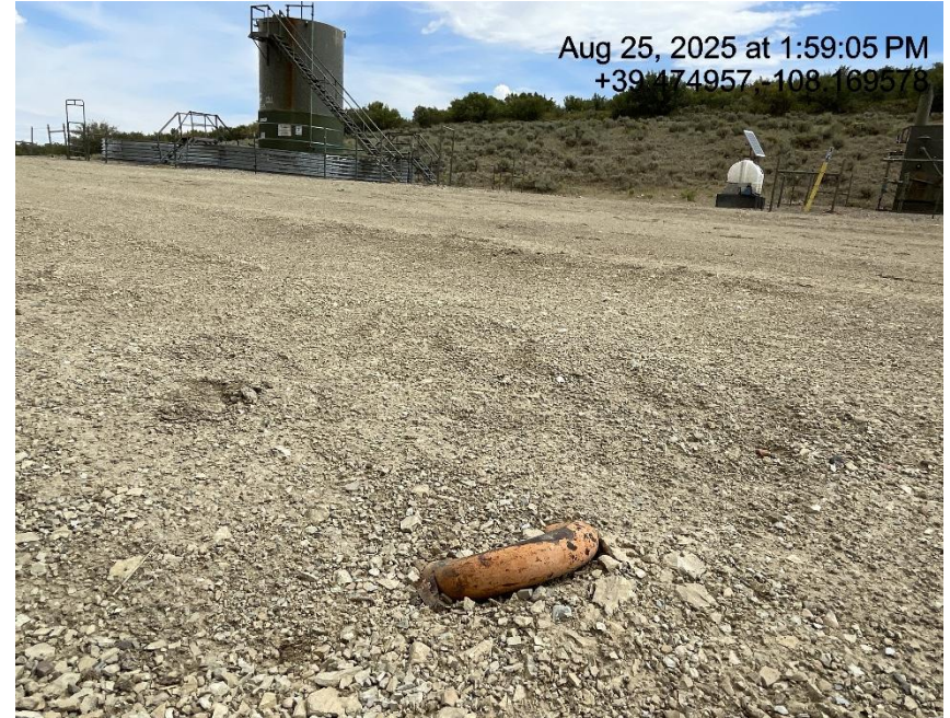
Photo # 4025 Same unmarked deadman
