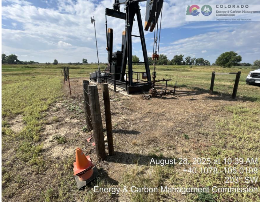
Torn down fence
