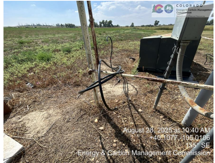
Exposed wires
