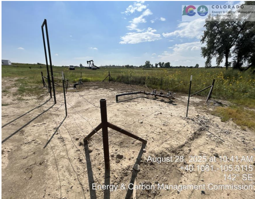
Removed overgrown vegetation
