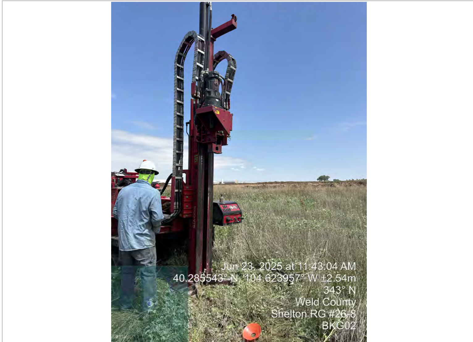
BKG02 Location: View North
