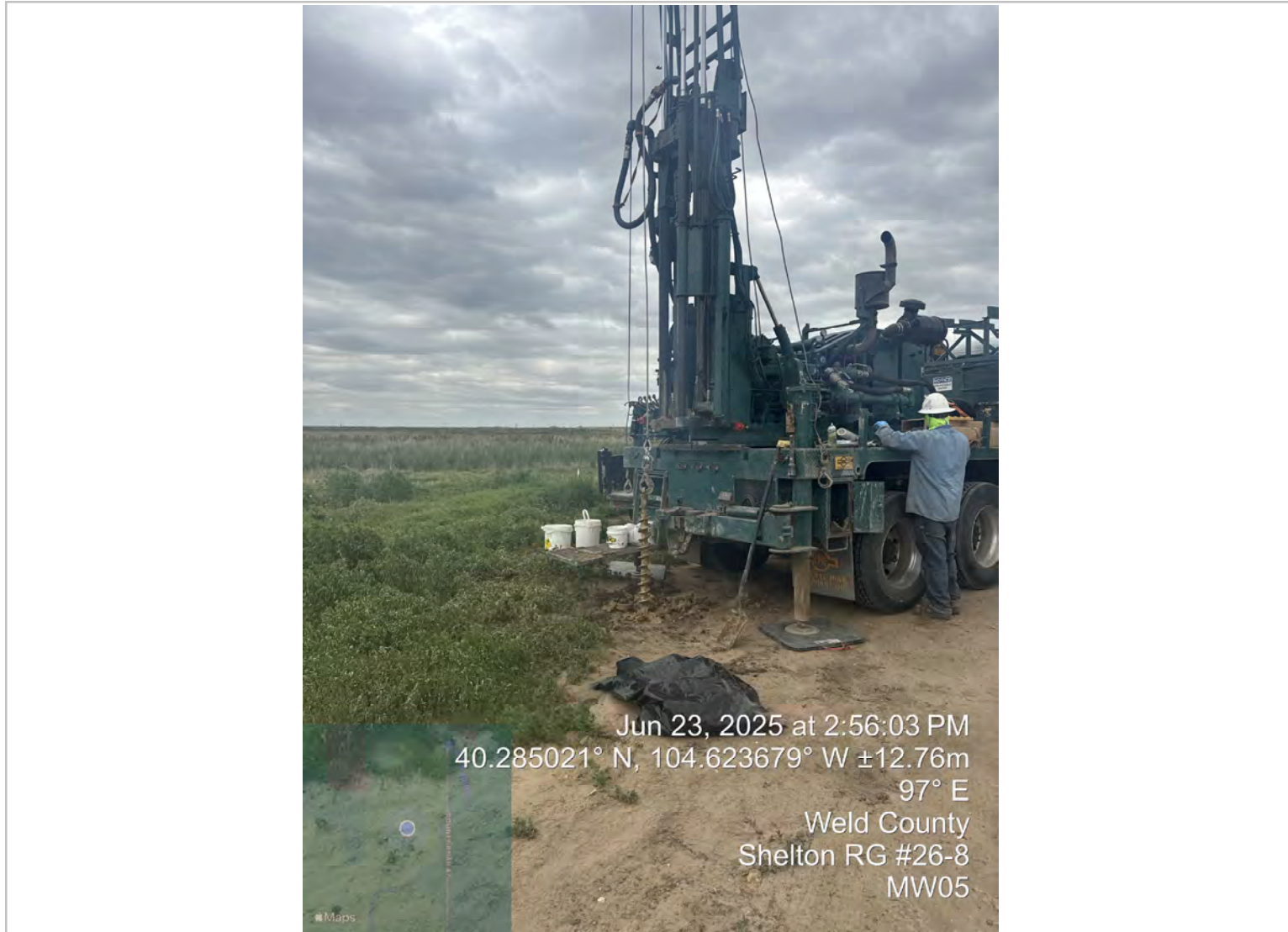
MW05 Location: View Northeast
