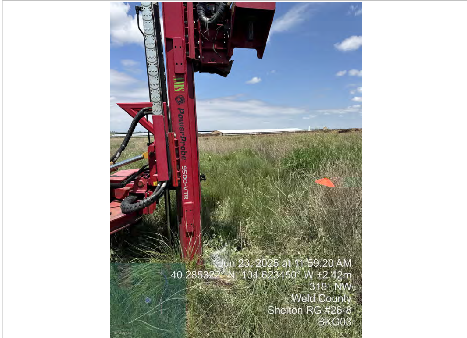
BKG03 Location: View Northwest
