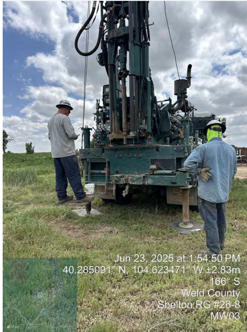
MW03 Location: View South
