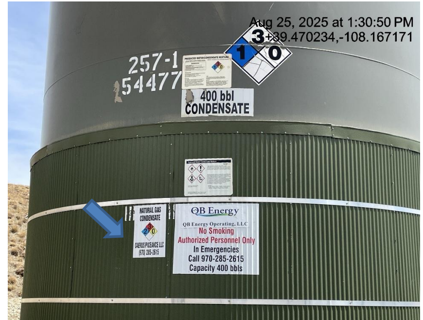
Photo # 3949 Tank label has previous operators name
