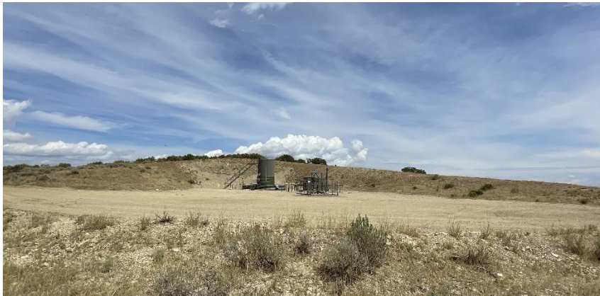
South West corner of location.
