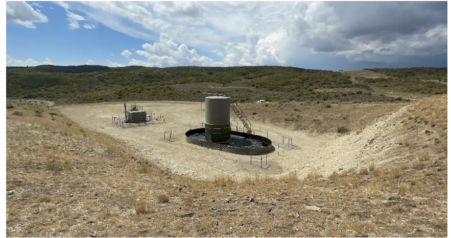
North East corner of location.
