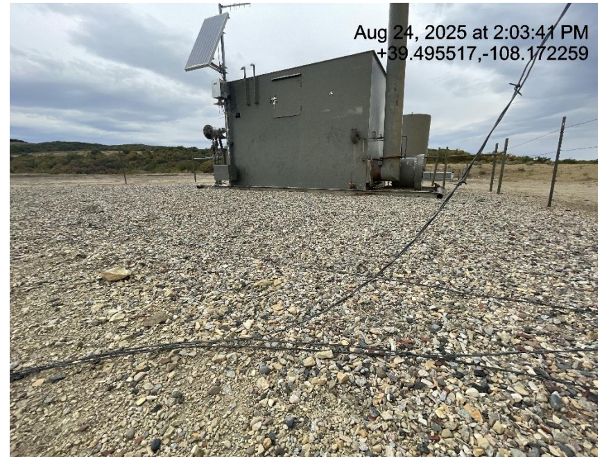
Photo # 3141 Barbed wire fence needs maintenance/wildlife & personnel hazard
