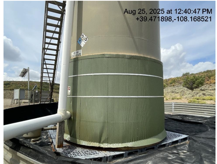
Photo # 3726 Tank lacks required labeling
