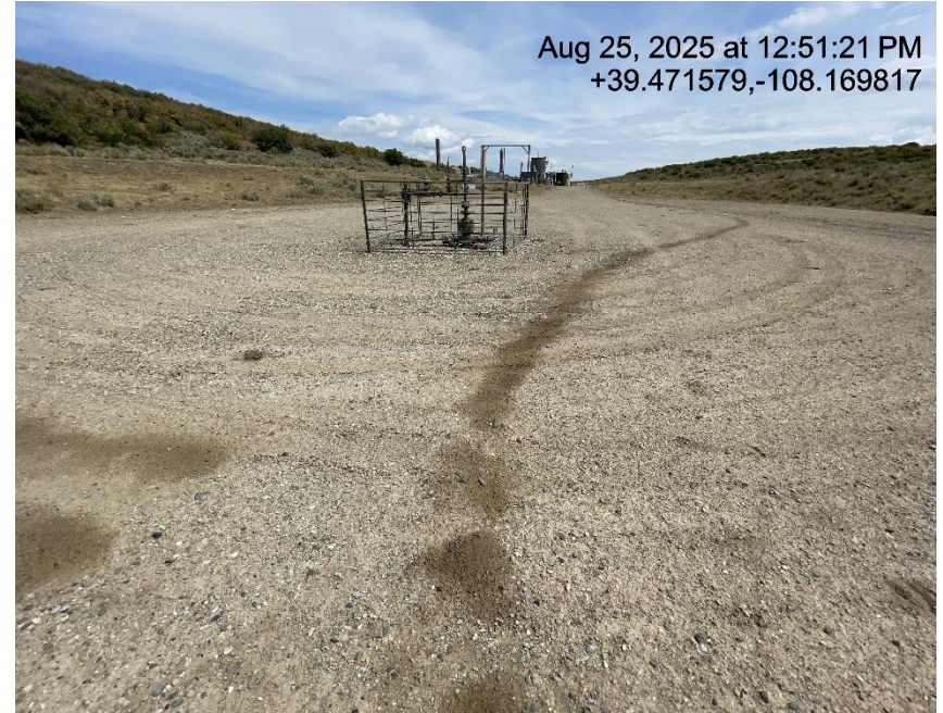
Photo # 3738 Stained soils
