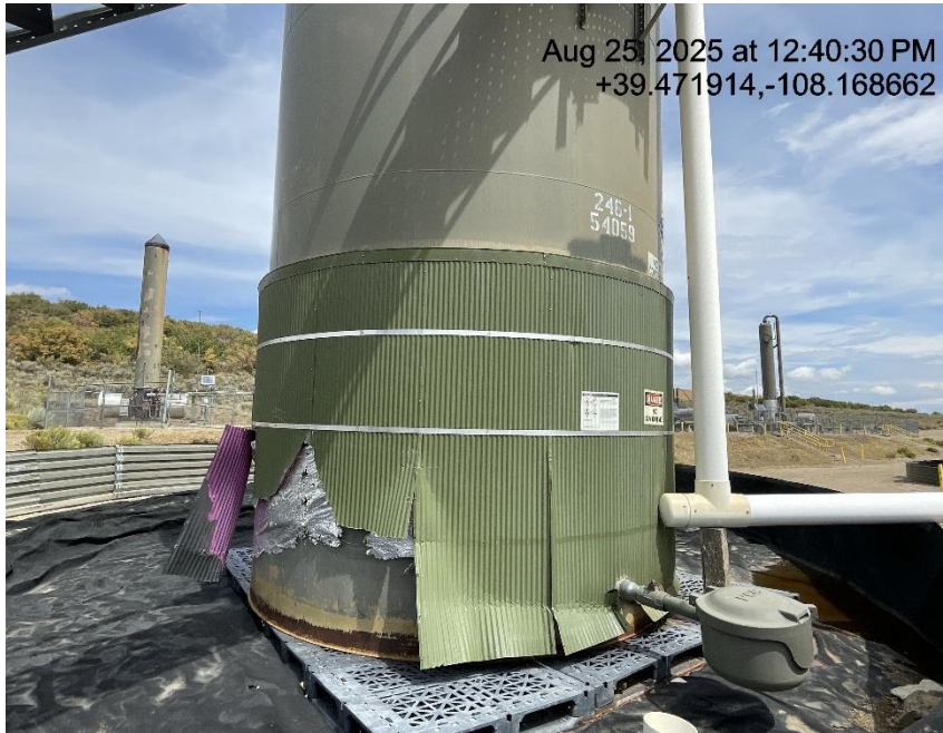
Photo # 3725 Tank lacks required labeling
