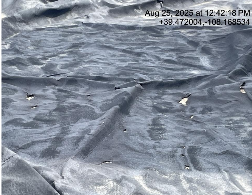
Photo # 3731 Holes in liner/liner needs maintenance
