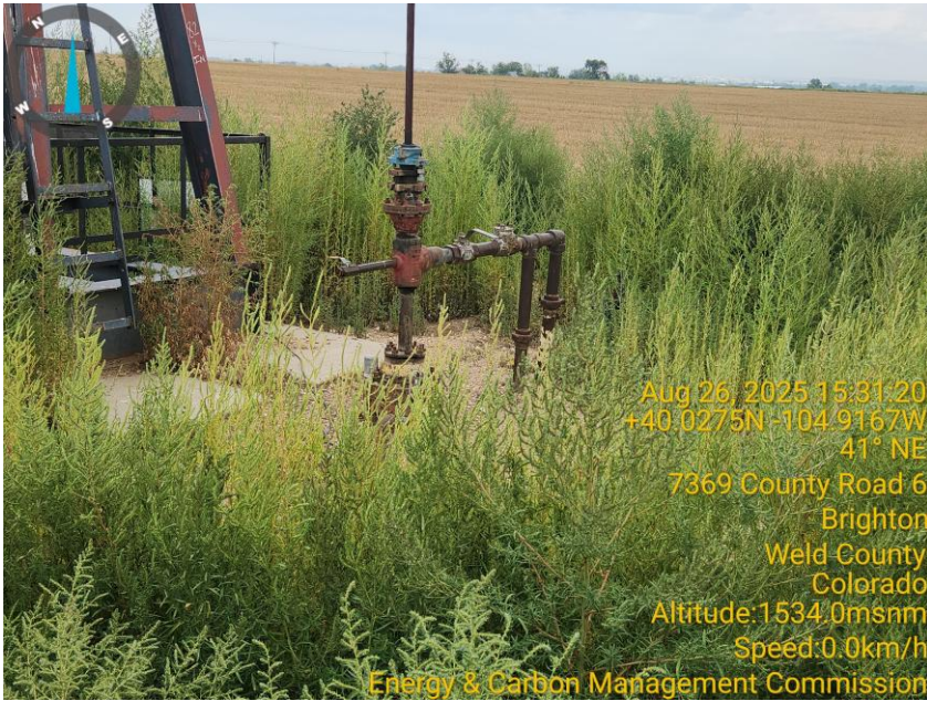
Photo 3 Wellhead in vegetation.
