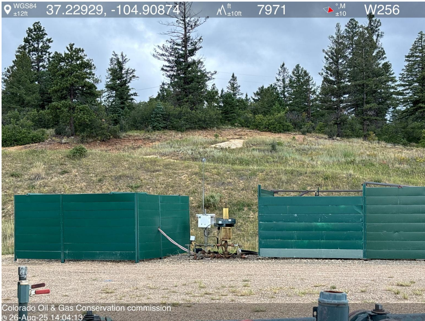
PHOTO 4: TR WELLHEAD AND EQUIPMENT.
