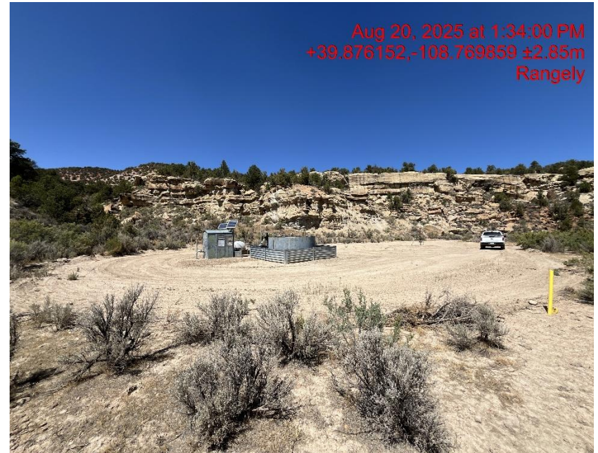
Photo # 2387 SE corner of location
