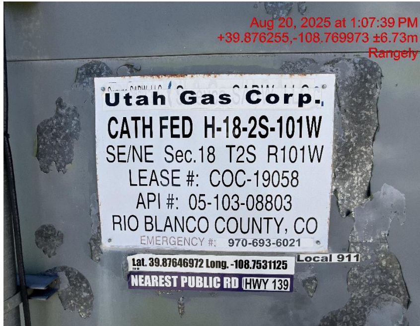
Photo # 2358 Battery sign lacks required information/not in compliance with CECMC rules, also Lat/Long is inaccurate
