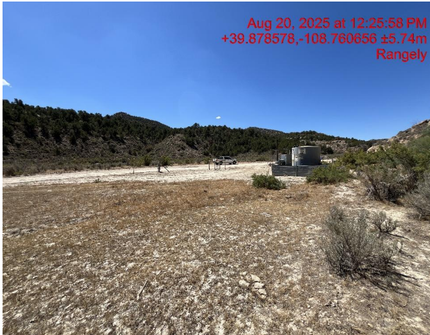
Photo # 2337 NE corner of location
