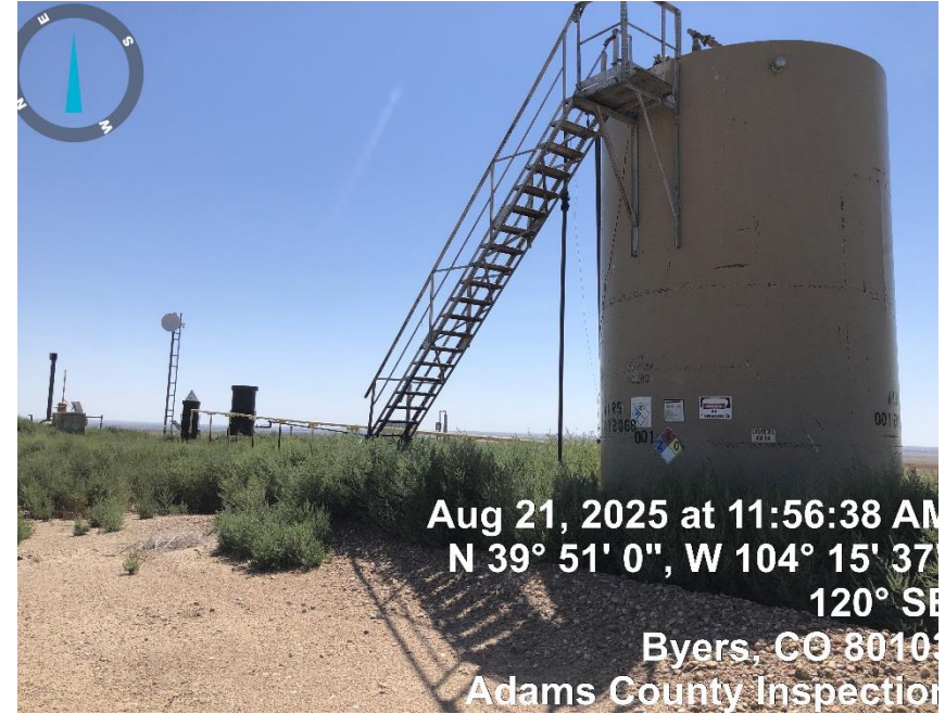
Photo#2 Production Tank/Separator/(2)ECDS/Gas Meter/ CA:Weeds uncontrolled throughout location
